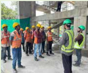
De-shuttering and Barricading
