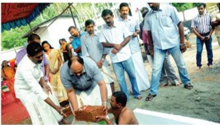
Another Milestone: Asset Homes Managing Director V Sunil Kumar and Executive Director K Anil Varma laying the foundation stone of Asset Darshan, the 50 th housing project of Asset Homes at the project site in Guruvayoor.
