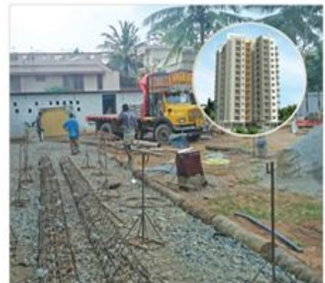
Construction in Progress at Asset Lineage, Thiruvananthapuram
