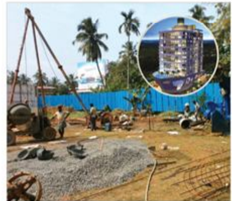
Construction in Progress at Asset Anchorage, Thrissur
